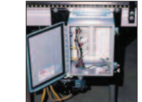
Electronics: Typical pre-wiring of components to local junction boxes
