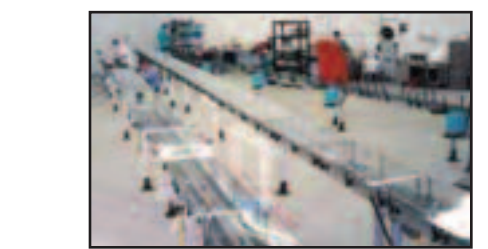
Automotive: Complete pre-assembly of inter-building transport lines
